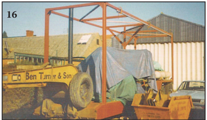
Work on converting the trailer into a curtain sider had begun
